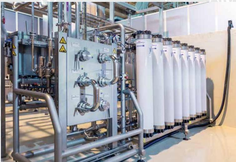
For water treatment, the plant uses a Krones Hydronic UF, in which the water is ultra-filtered using start-of-the-art membrane technology and hollow fibres.
